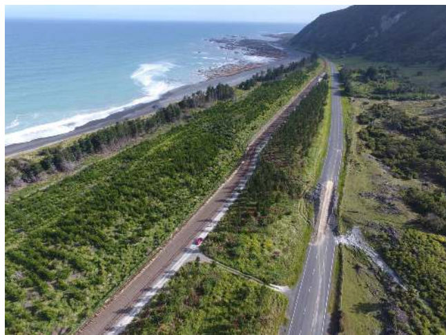
Figure 2. Damage to State Highway 1 and the railway track near Kaikōura (GeoNet, 2016; photo credit Julian Thomson).
