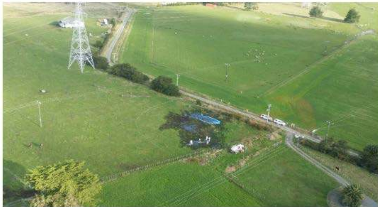
Photo of Petroleum Leak
