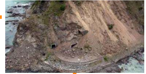
Event Occurs - Building and Infrastructure Damage
